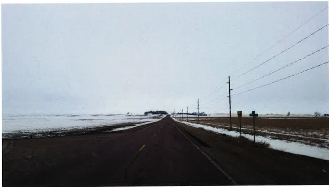
A22/170th Street pavement
